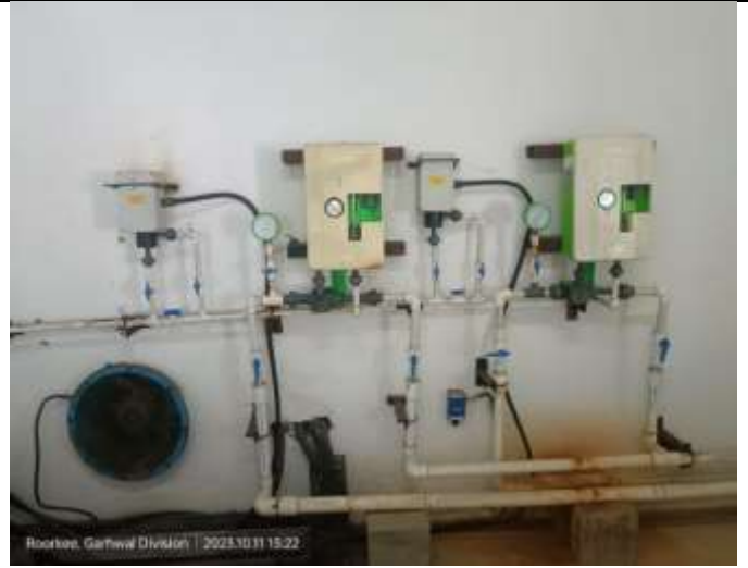
Fig 6: Gas chlorinator
