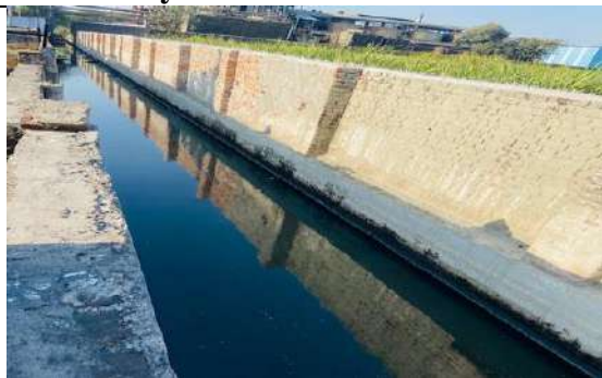
Photo 19: Laksar drain passing from the premises
