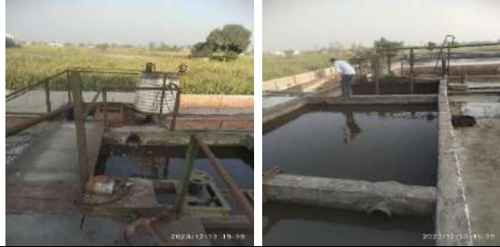
Photo 13: Alum dosing and tube settler
