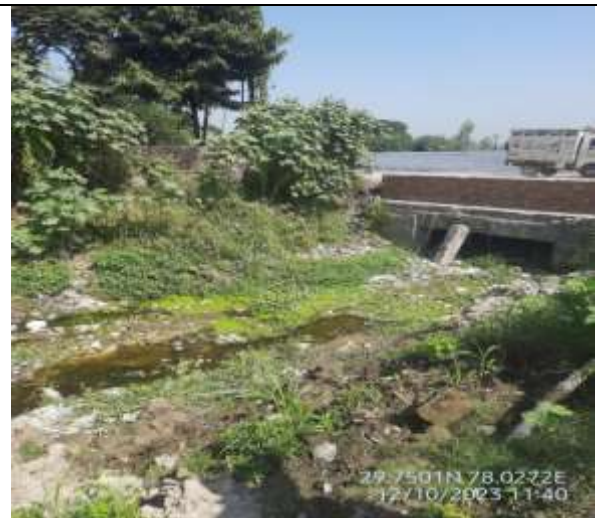
Figure 29: Solid waste dumped along Laksar drain
