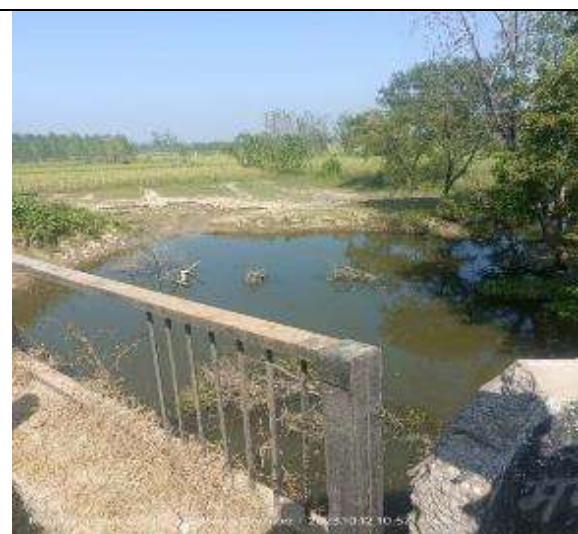
Figure 36: Hadwa drain at Roorkee- Laksar road, u/s of Laksar
