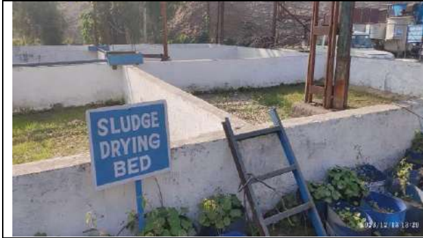
Pic.-15.SRS outlet discharge to ETP inlet channel
