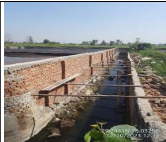
Figure 30: Laksar drain near lagoons of the unit
