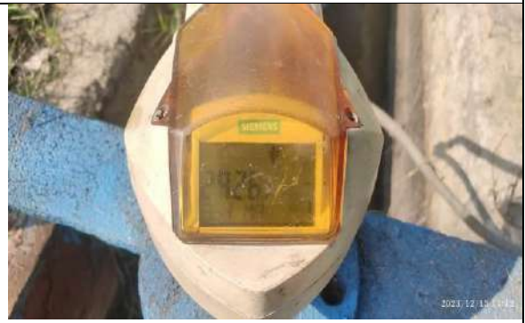
Pic.-18.Imbibition water flow meter
