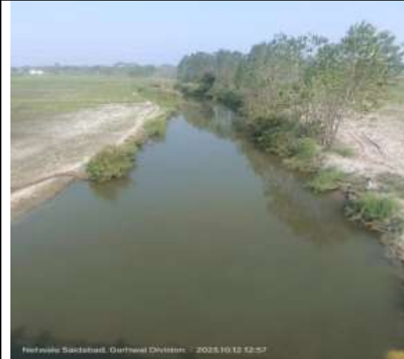
Figure 16: River Banganga at Laksar-Balawali Marg bridge, d/s of Laksar
