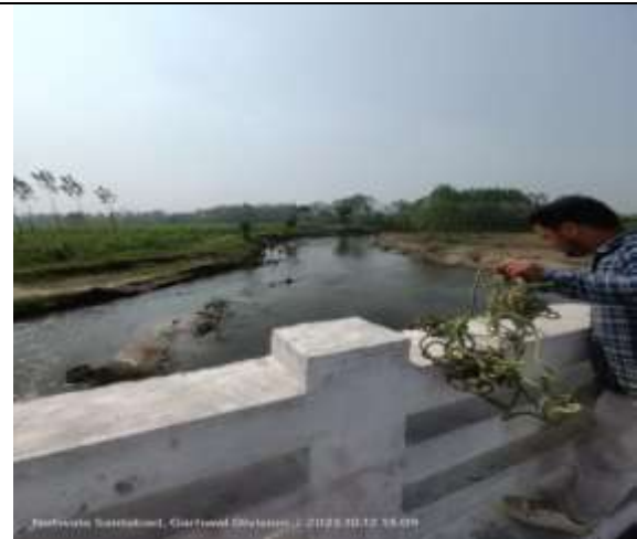
Figure 23: River Solani downstream of Roorkee at bridge on National Highway
