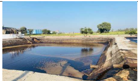
Photo 20: Lagoon for storage of conc. spent wash
