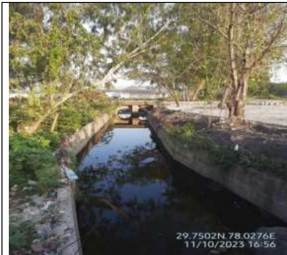
Figure 28: Laksar drain upstream of unit
