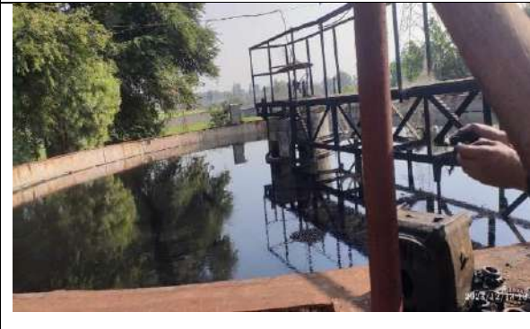
Pic.-10.Secondary clarifier
