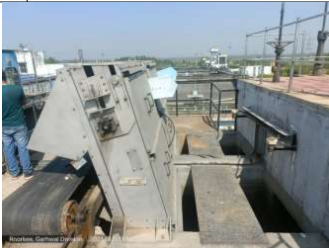
Fig 1: STP inlet screen
